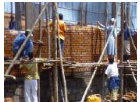
Construction work in Kibeho: The new convent of the Pallottine Sisters.
