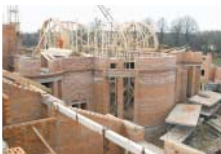
Spring 2003. The walls rise up, the seminary takes shape.
